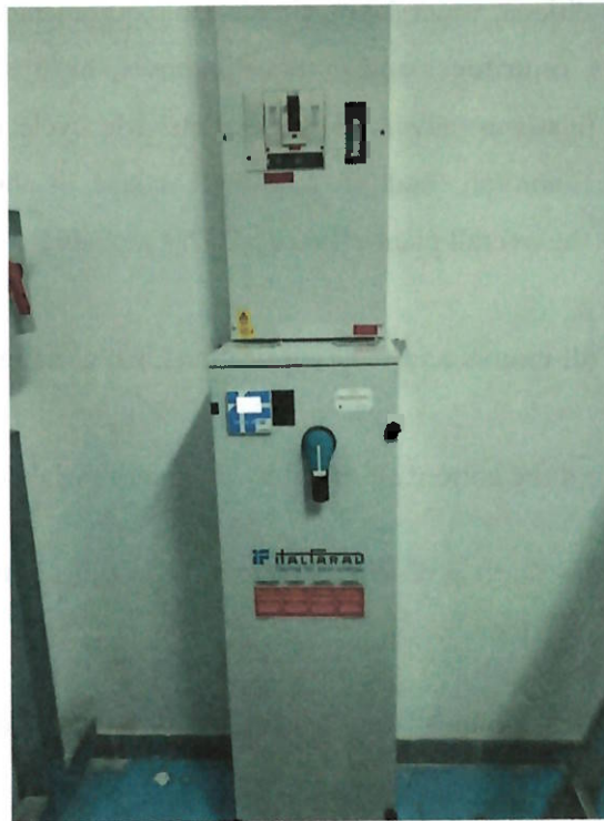
Figure 14. Power factor corrector
